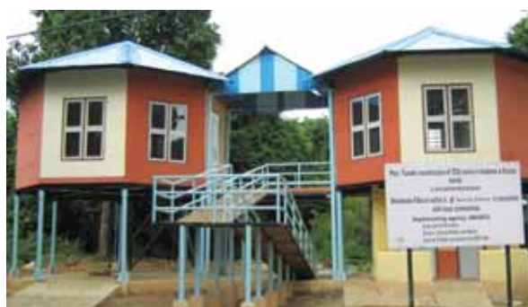
One of the new children's centres, built on stilts to avoid flooding
